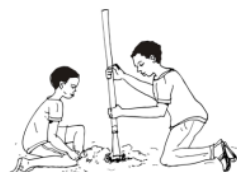
1. Dig two small holes about 2 feet apart
