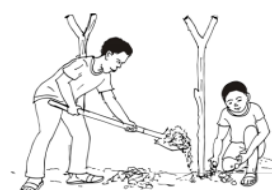
3. Fill each hole with sand and stone to pack the sticks tightly so that they don't move
